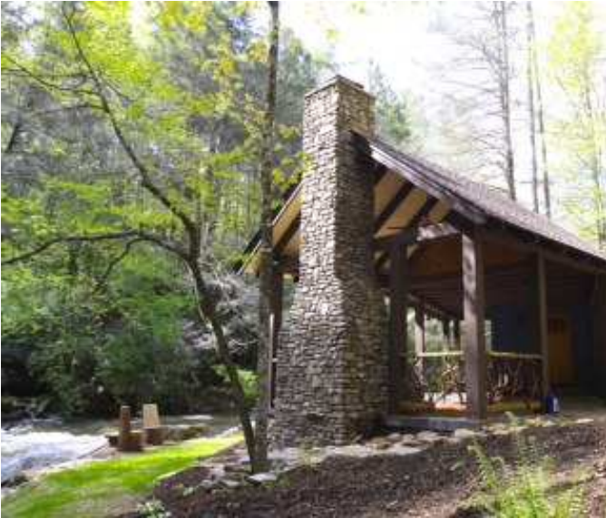
Side shot of the pavilion with the river on the left.
