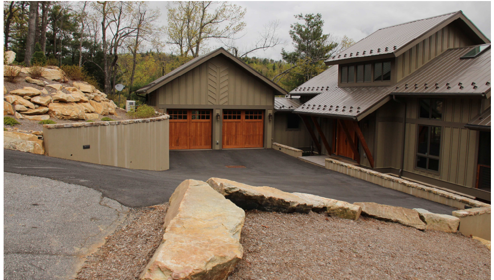
Due to having a retaining wall in the front, as well as mulch and rock landscaping with no downed dead fuel or trees and shrubs immediately next to the home, Grady & Kathleen Nance's home on Mountain Maple Drive is one example of good landscaping that is "firewise."
